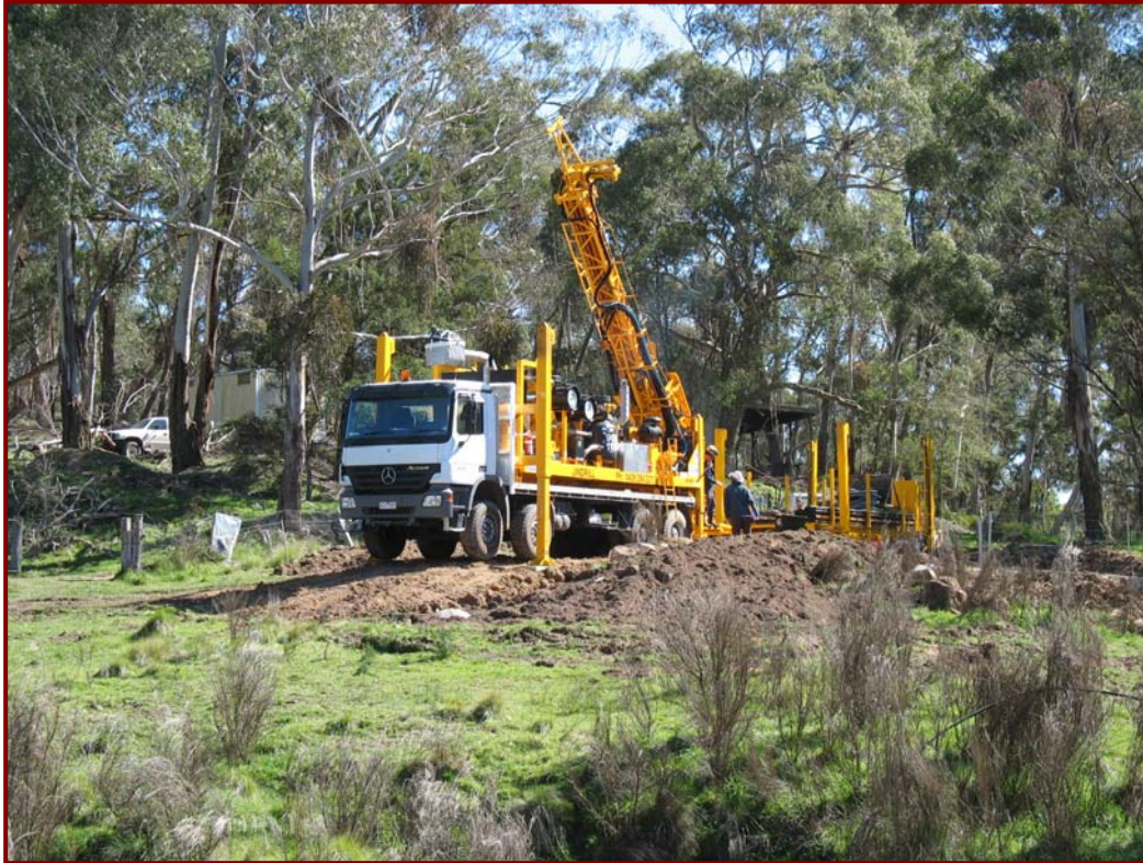
Figure 2: Drilling rig working at Dargues Reef
