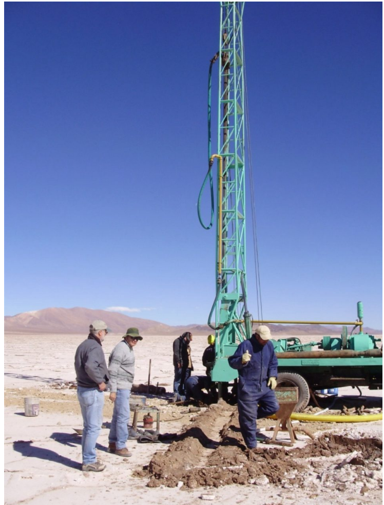
Drilling the first water bore
