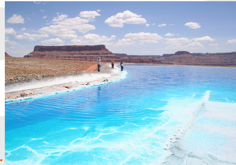
Potash evaporation ponds owned by the Intrepid Potash Co., Dead Horse Point, Utah.
