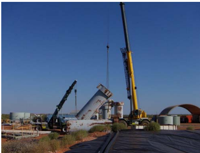
Crane dismantling carbon columns from the Indee site
