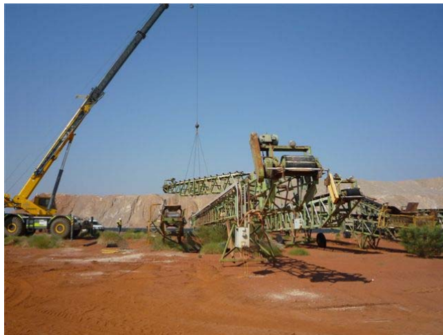
Dismantling grasshopper conveyors at Indee
