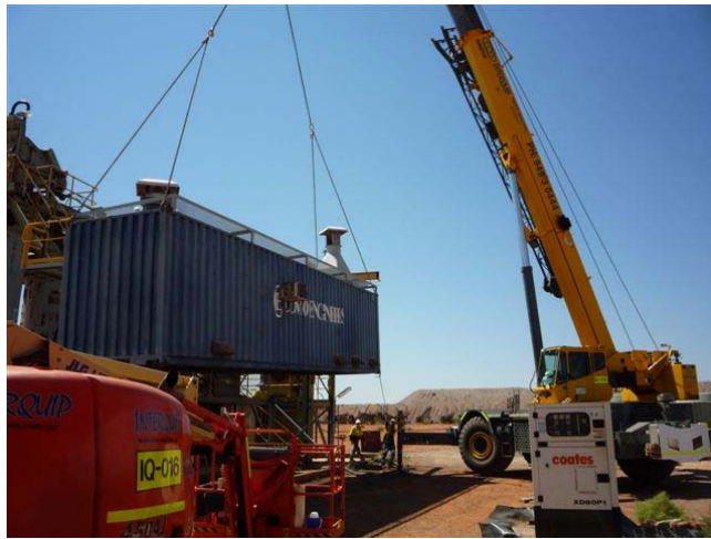
Crane removing the gold room from the Indee site
