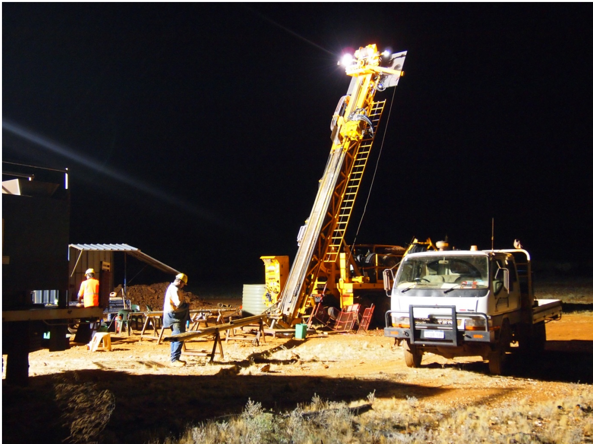
Figure 2 Diamond drilling of geotechnical holes at Burnakura
