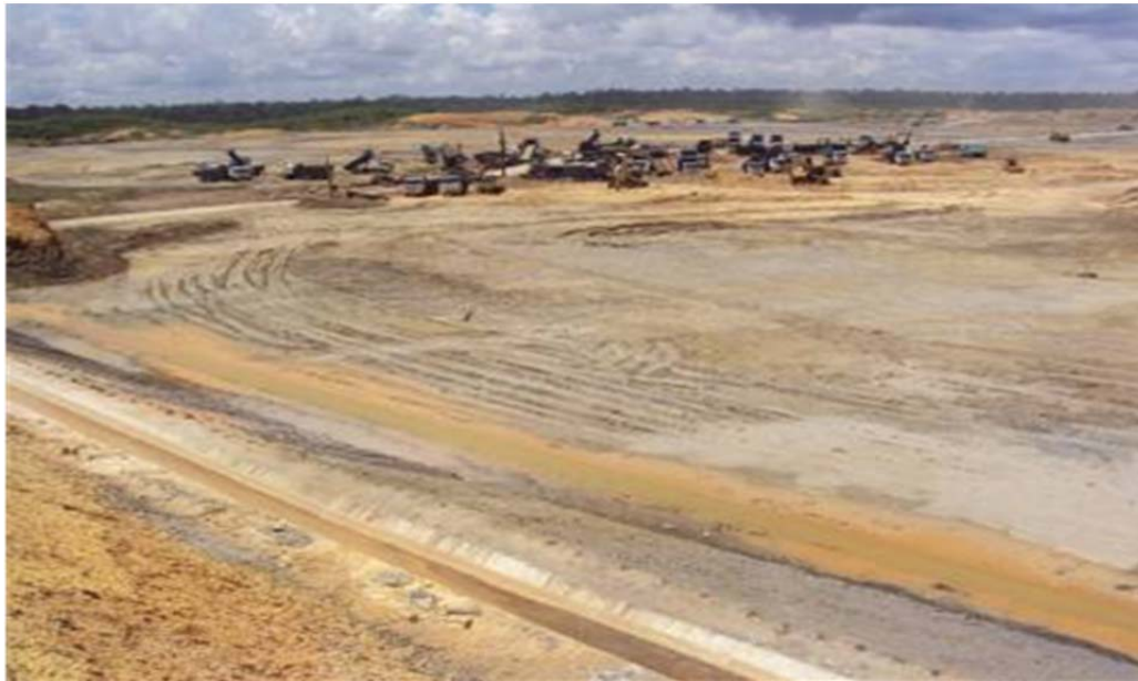
Earthworks at the OM Samalaju Site
