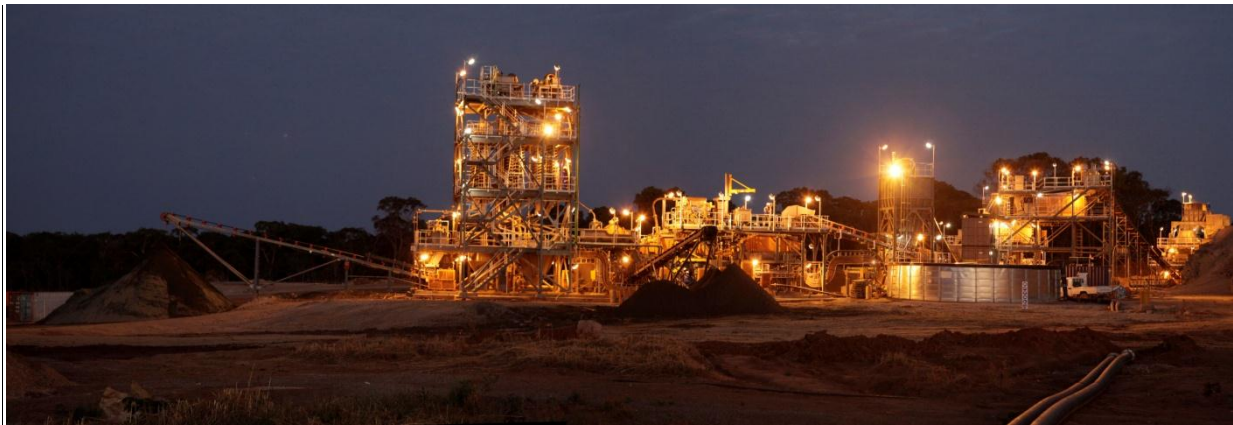
Kipoi HMS Plant
