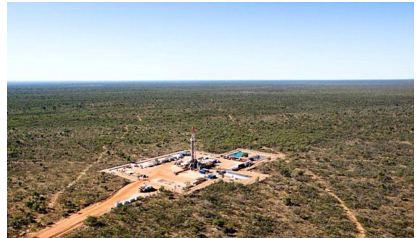
Ensign Rig#32 drilling Yulleroo-3
