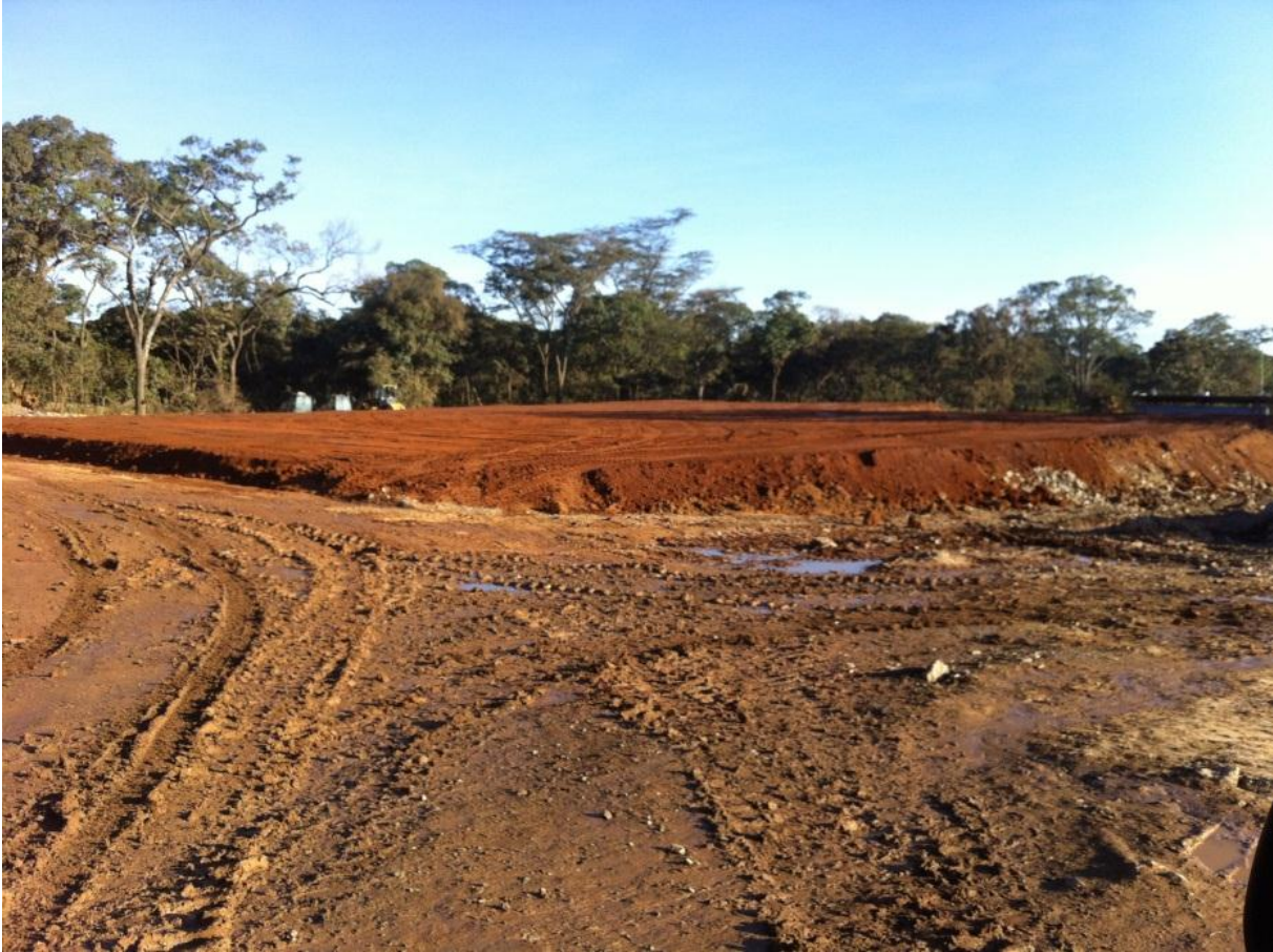
Completed site work for the electrical sub-station at Kipoi
