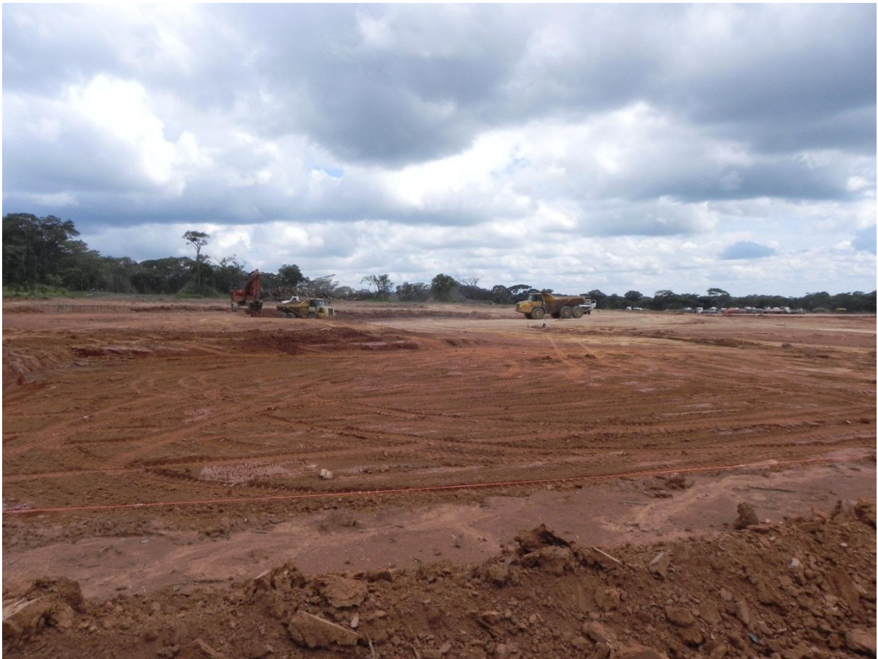
Site clearing for the SXEW plant
