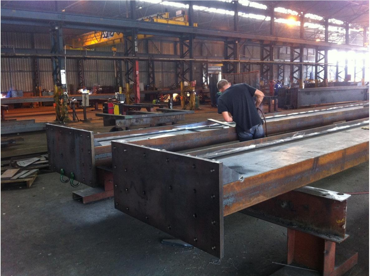
Fabrication of steel work for the EW tankhouse
