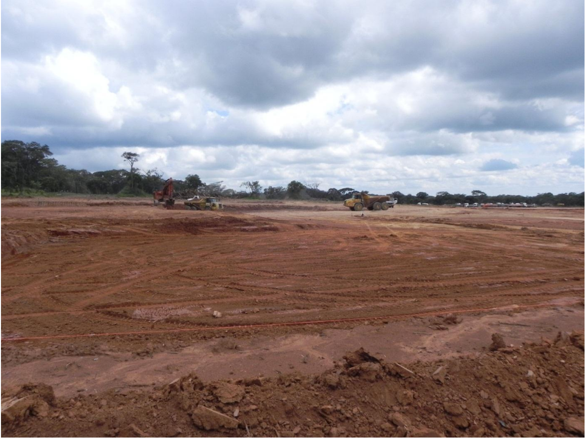
Site clearing for the SXEW plant
