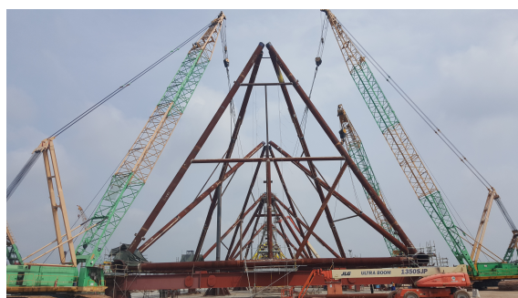
Figure 2 Ophir Jacket Construction
