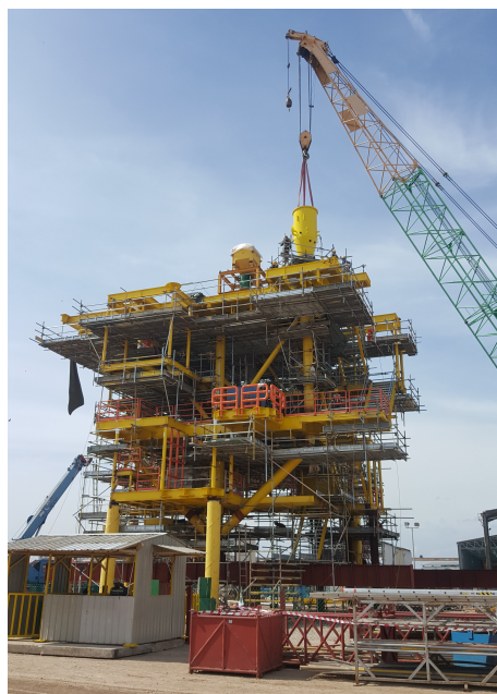
Figure 3 Ophir Topsides in Progress
